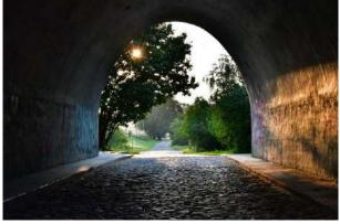
**TUNNEL AT THE BRIDGE ACROSS THE DAUGAVA** The tunnel (43.04 m long) is one of the few parabolic monolithic reinforced concrete structures in Latvia that was built in the 1920-30s. The driveway still has the original cobblestone pavement.
